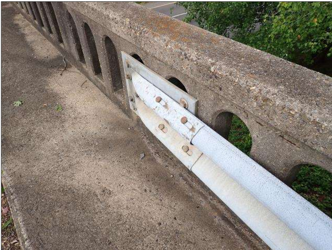
northwest guardrail attachment
