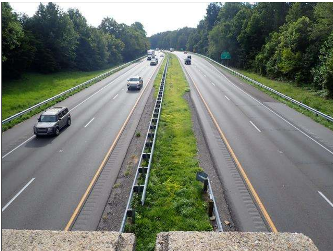
roadway looking east
