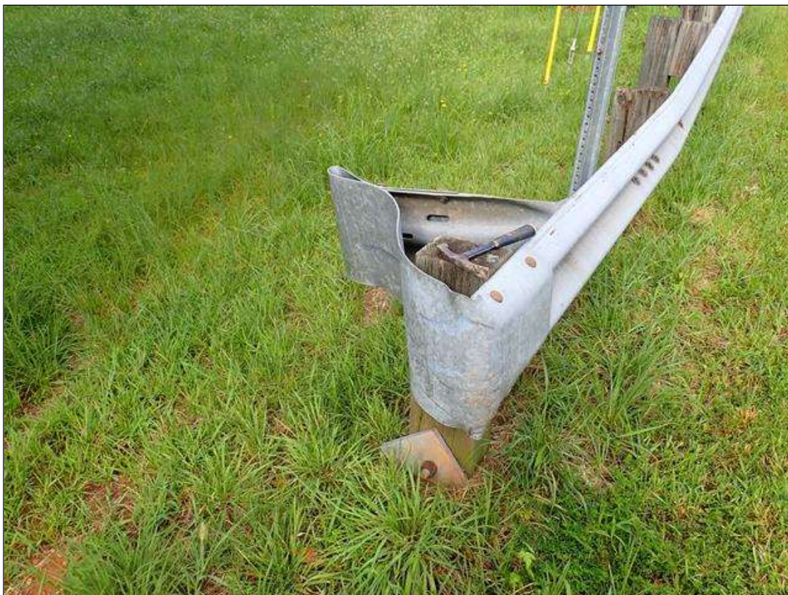
northeast guardrail termination
