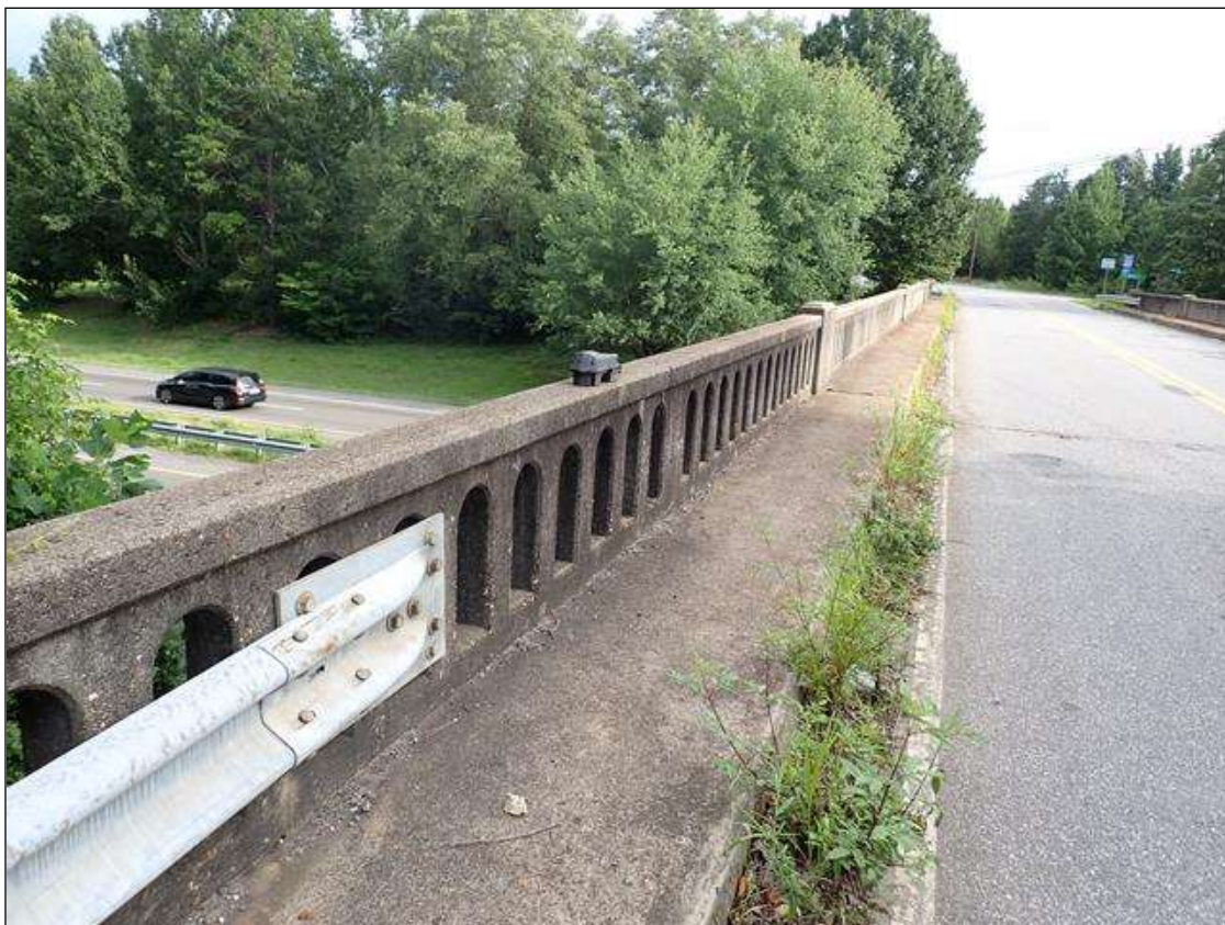
left bridge rail
