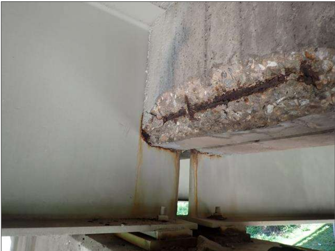
beams over bent 2
