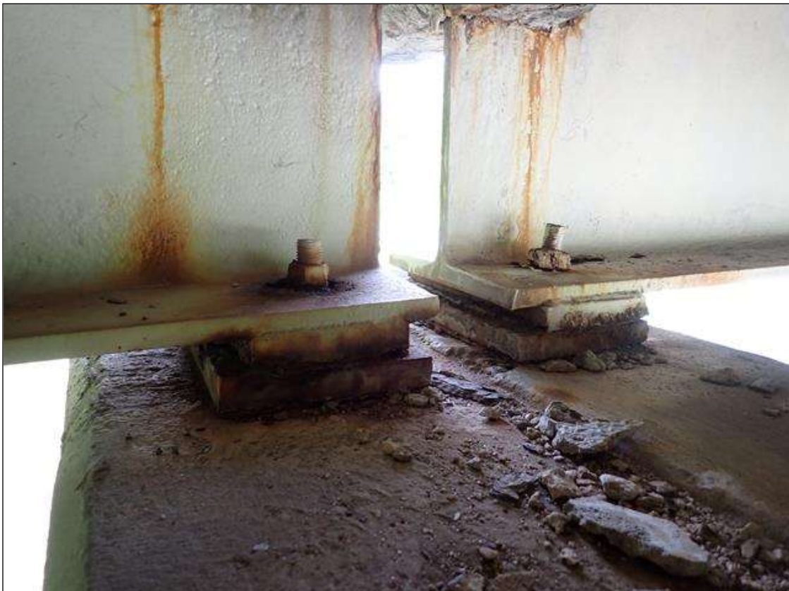
interior bearing assembly at bent 1 exterior beams (bent 3 similar)
