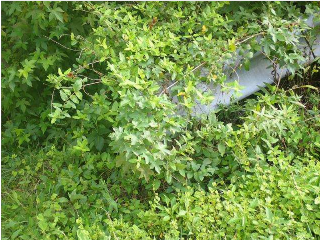
southwest guardrail termination
