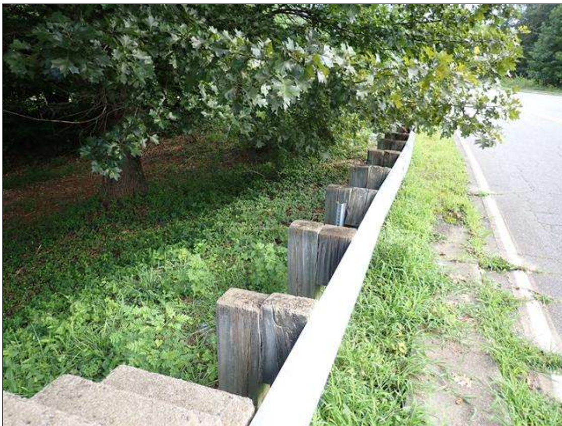
northwest guardrail transition
