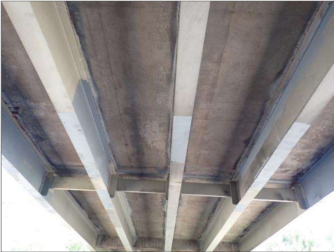
superstructure underside, span 2 (span 3 similar)
