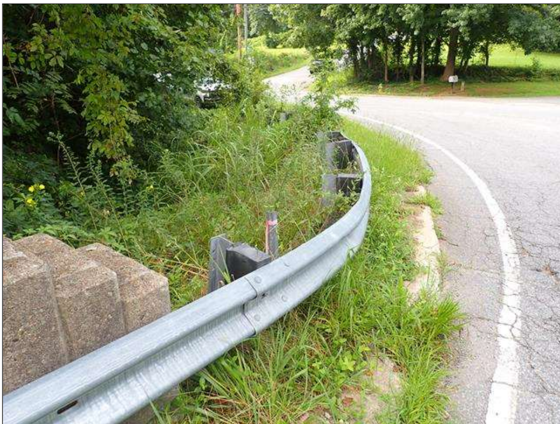
southeast guardrail transition
