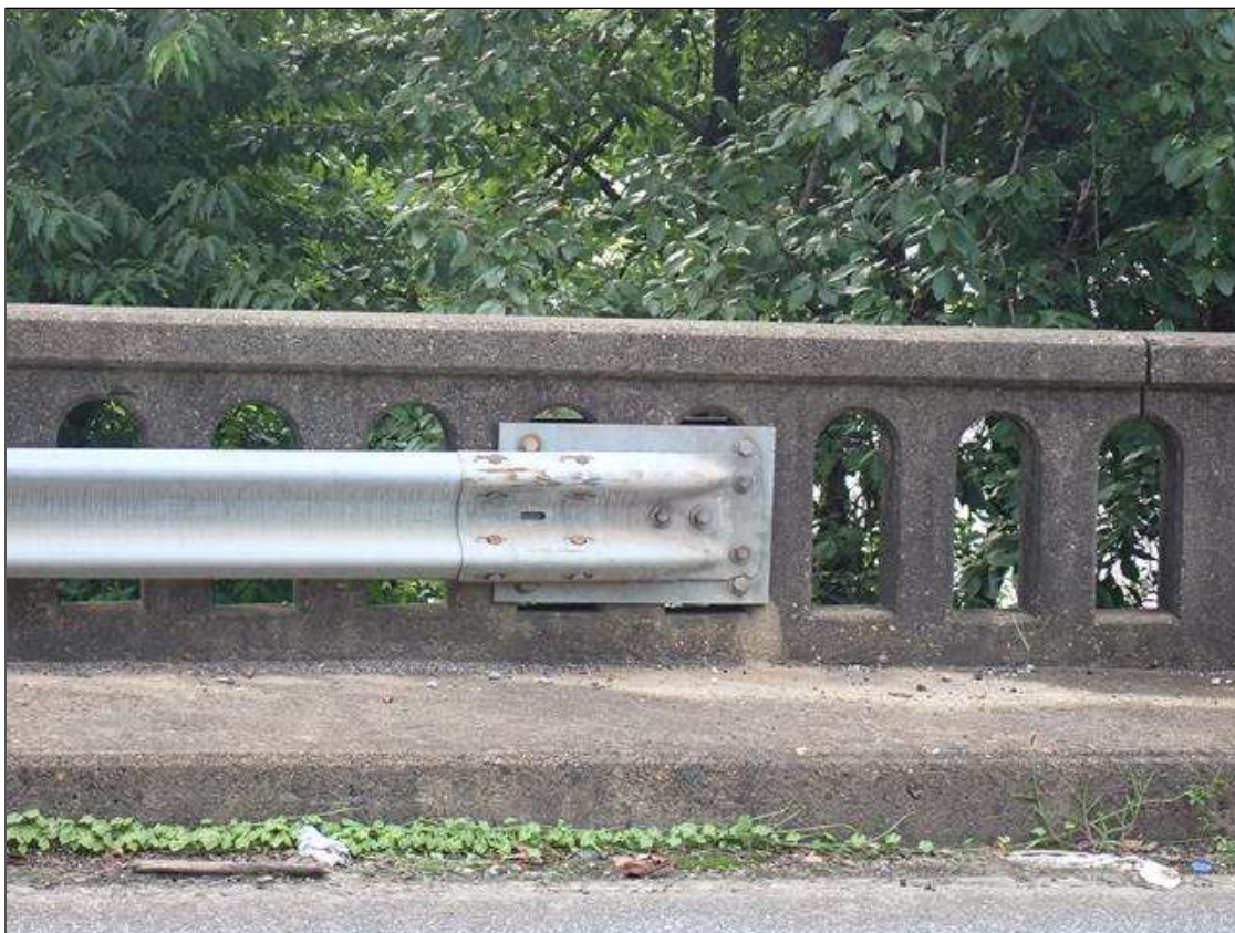
northeast guardrail attachment
