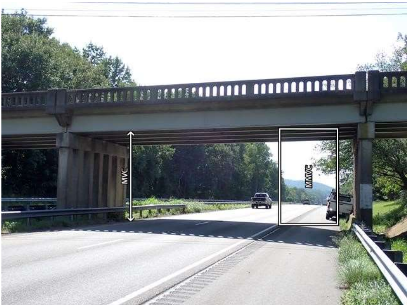
roadway under span 3, looking west (I-40 westbound)
