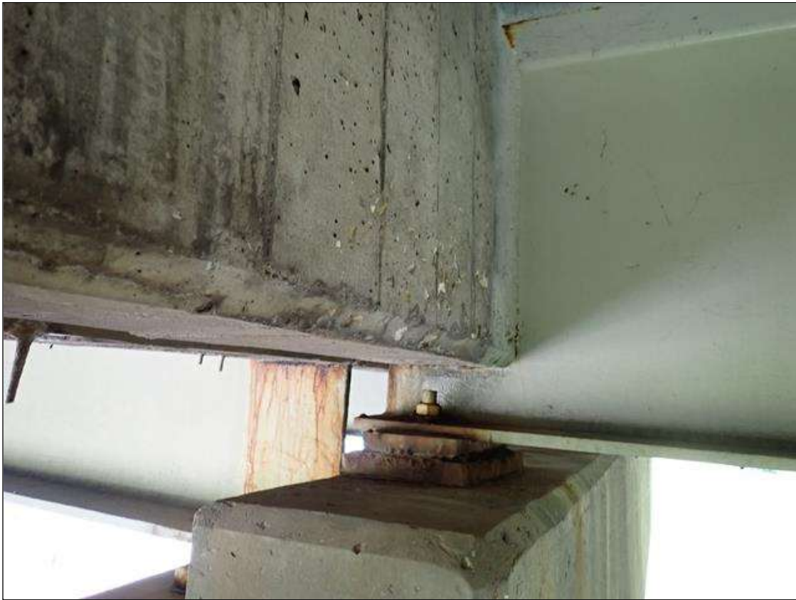
interior beams over bent 1 (bent 3 similar)
