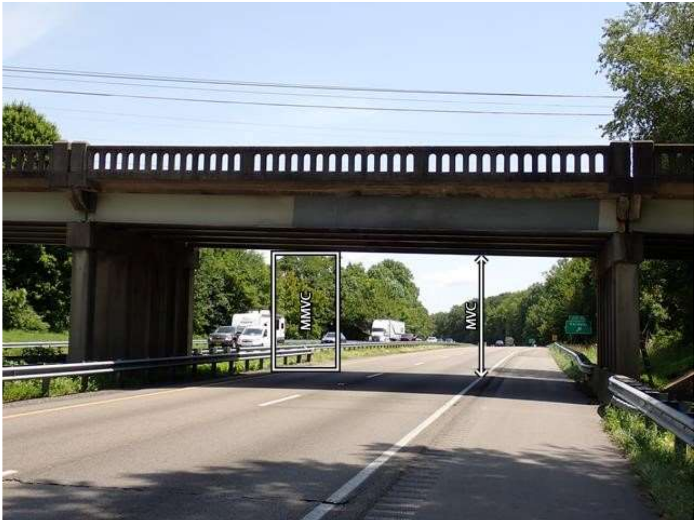
roadway under span 2, looking east (I-40 eastbound)
