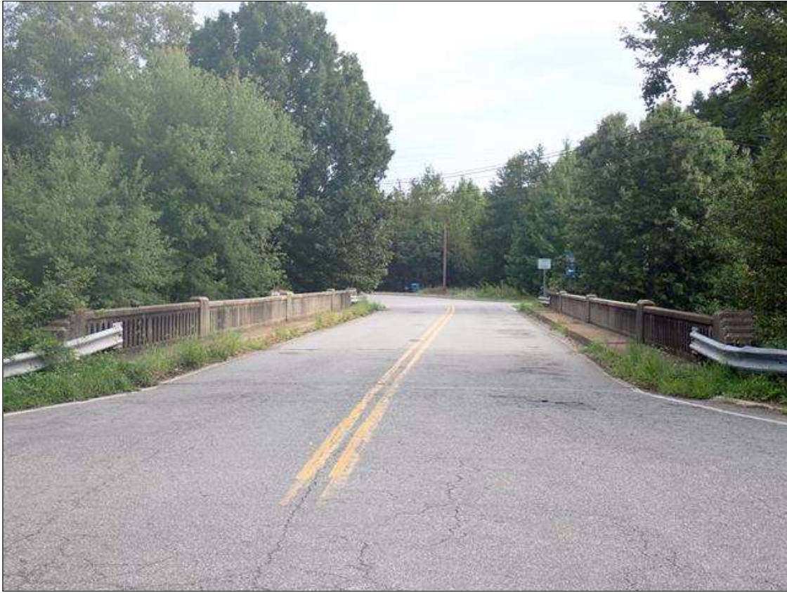
south approach looking north
