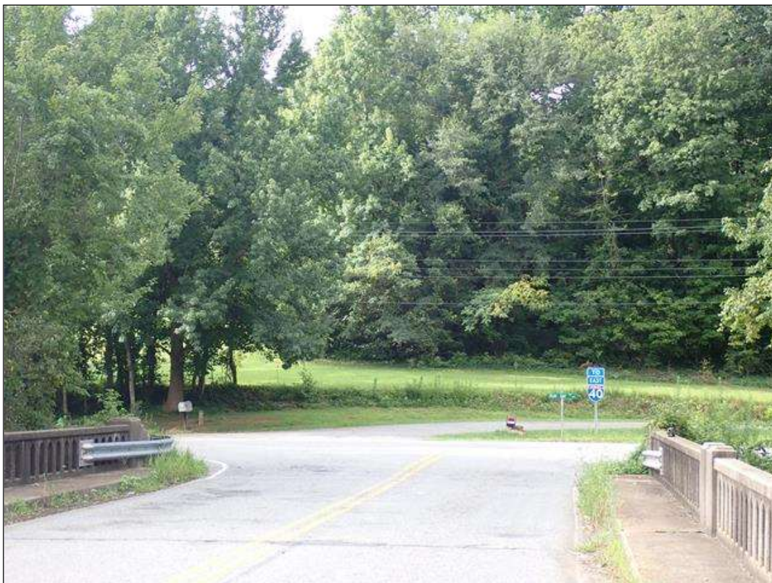
south approach looking south
