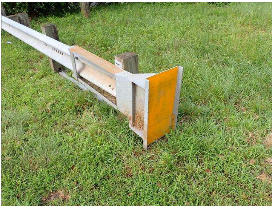
northwest guardrail termination
