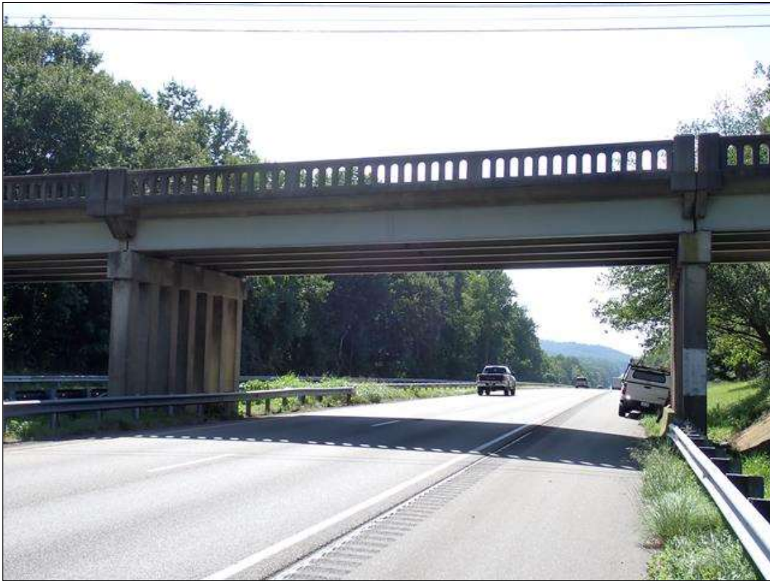
roadway under span 3, looking west (I-40 westbound)
