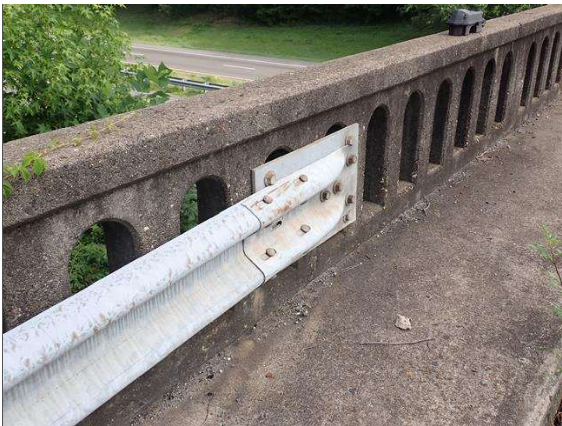
southwest guardrail attachment
