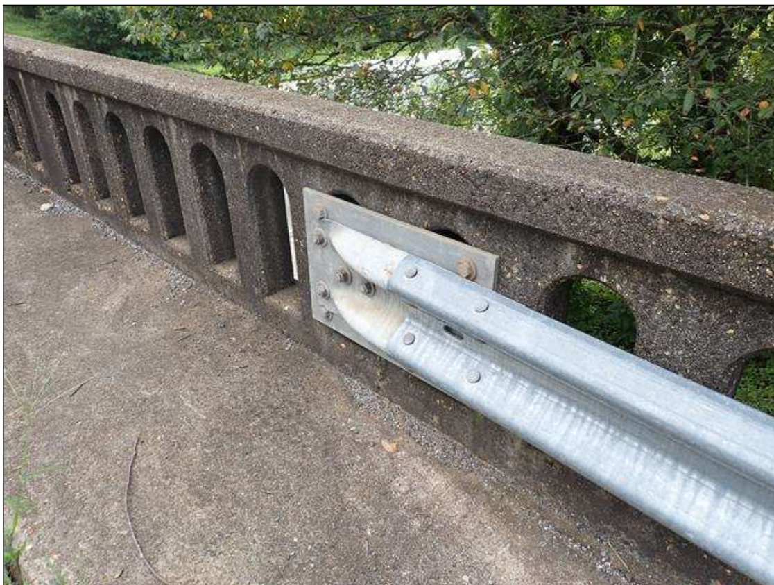
southeast guardrail attachment
