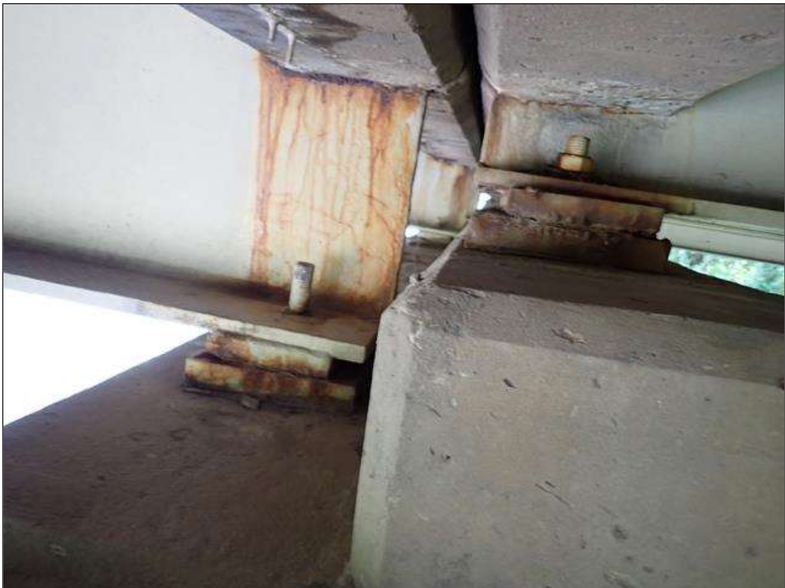
interior bearing assembly at bent 1 (bent 3 similar)
