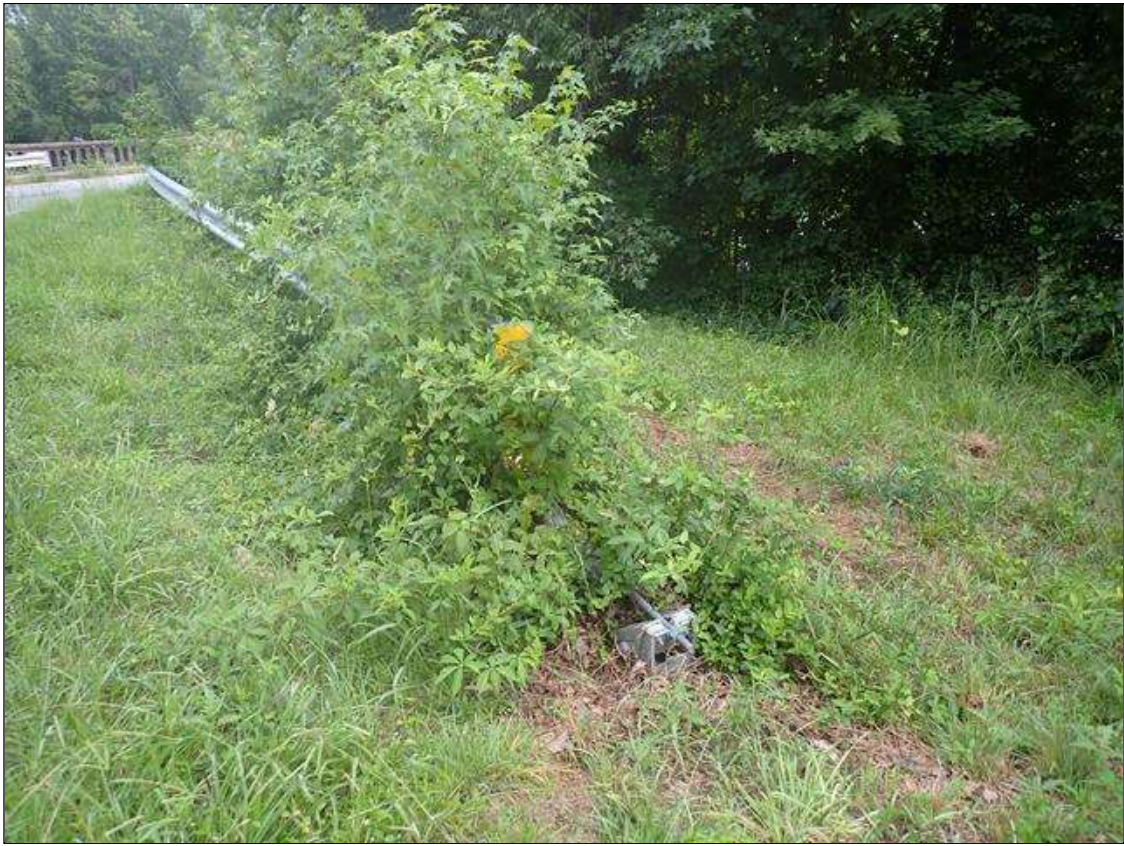
southeast guardrail termination
