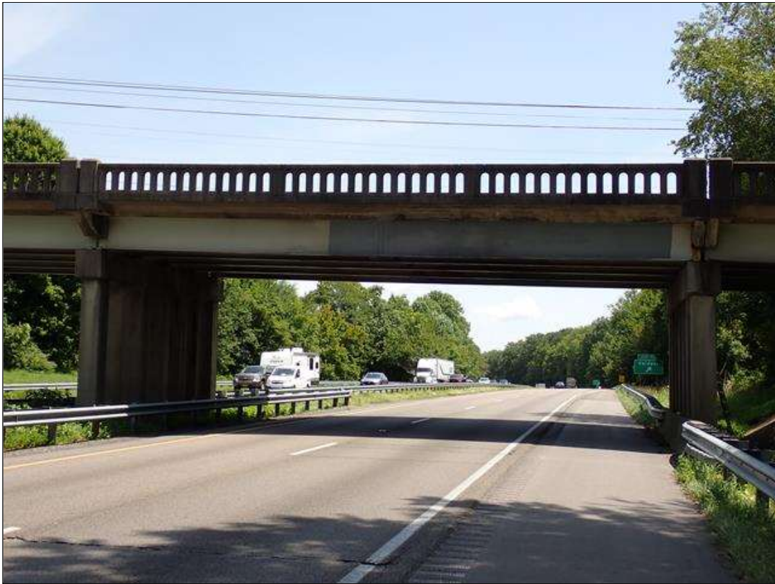
roadway under span 2, looking east (I-40 eastbound)
