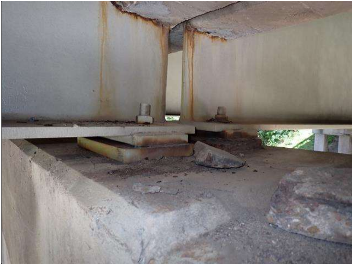
interior bearing assembly at bent 2
