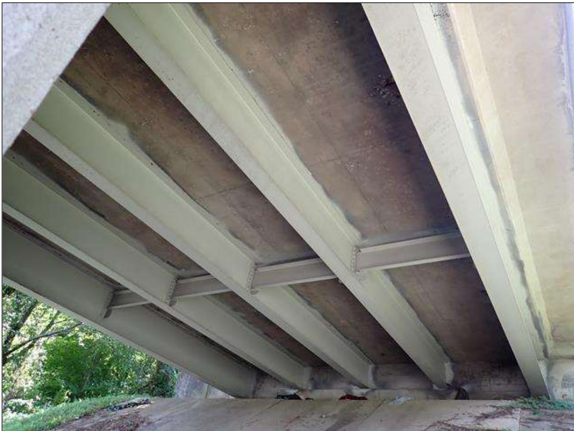
superstructure underside, span 1 (span 4 similar)
