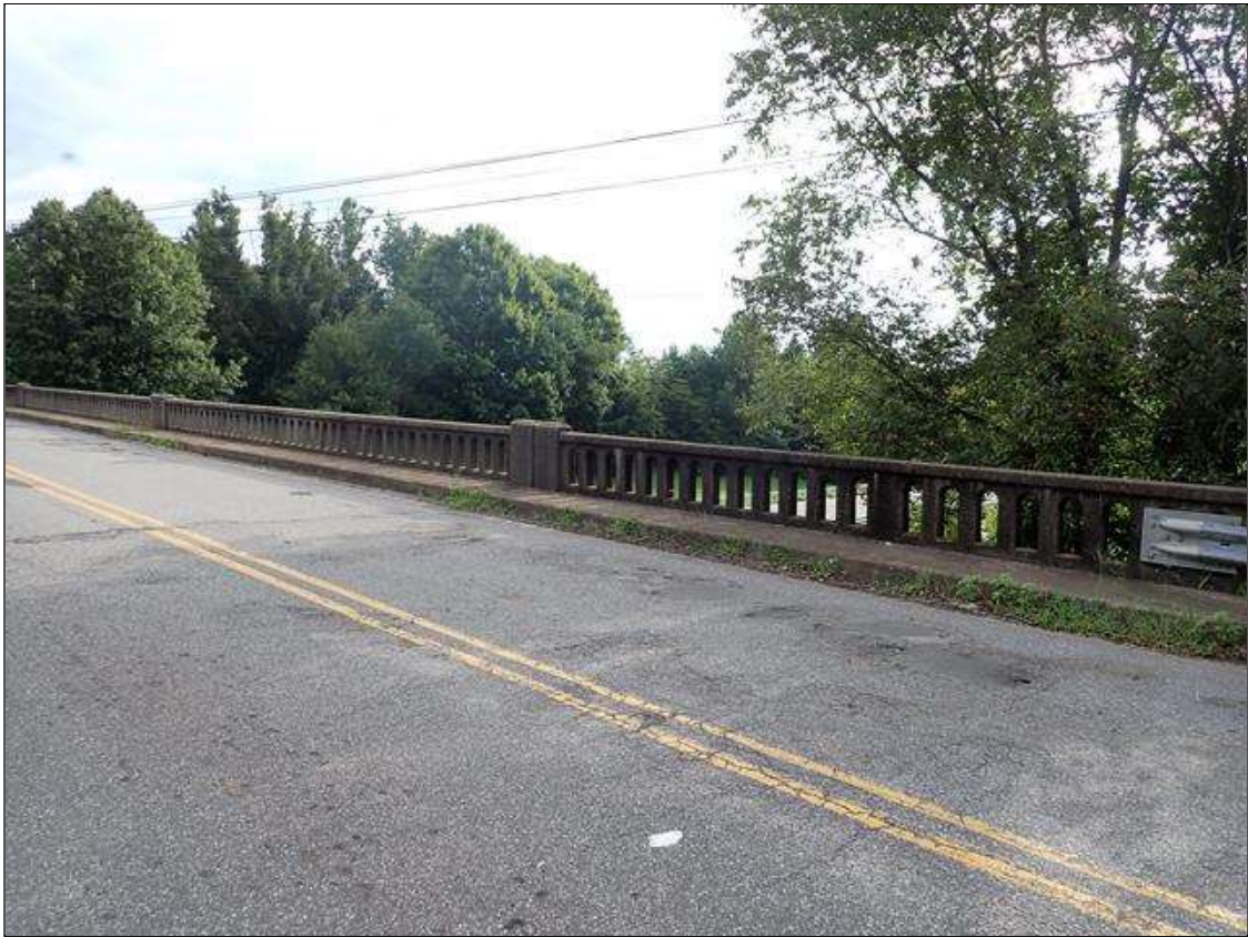
right bridge rail
