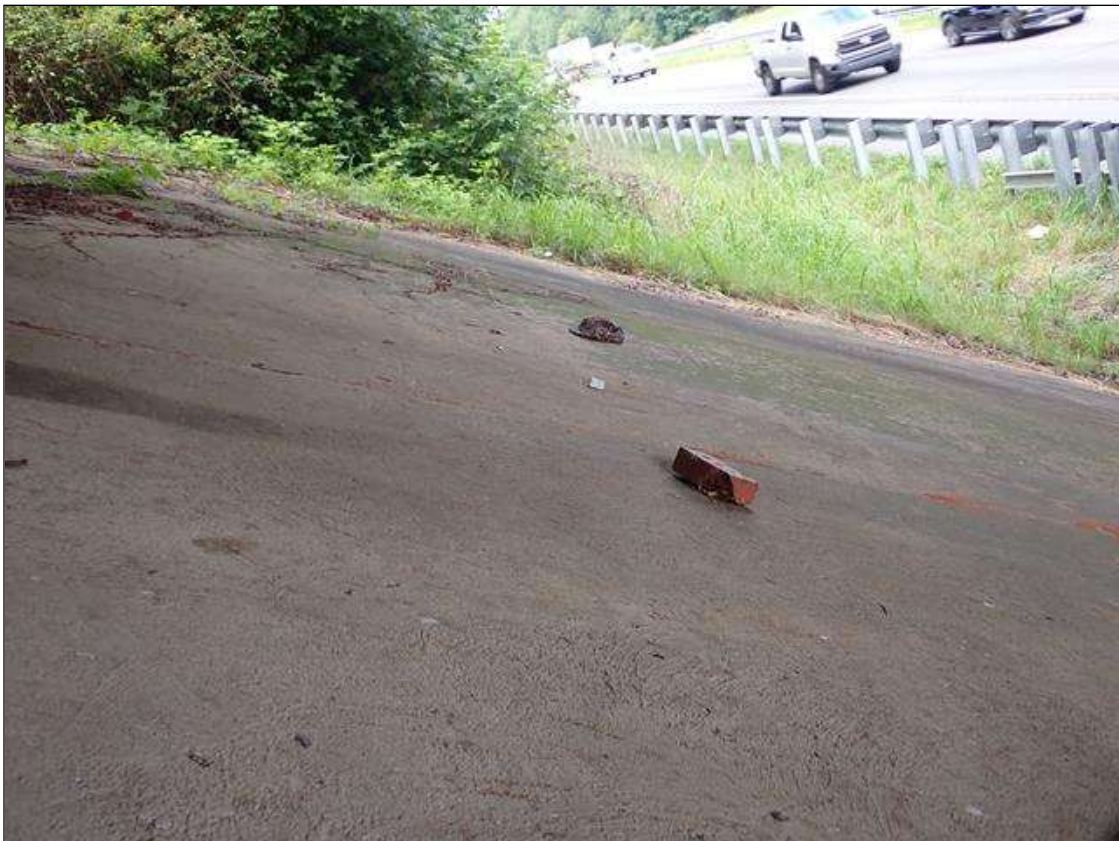
end bent 1 slope protection (end bent 2 slope protection similar)
