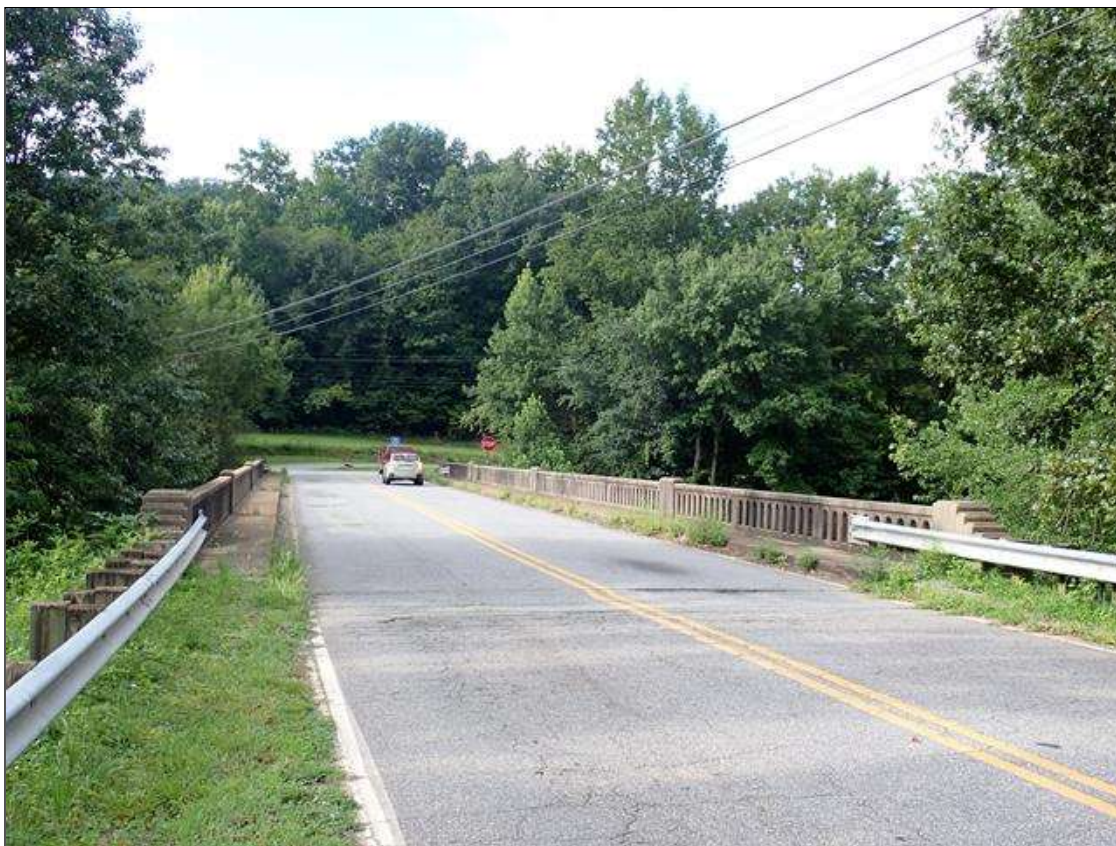
north approach looking south
